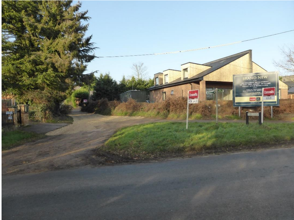
Figure 34 - Junction of Park Road with Heath Road
