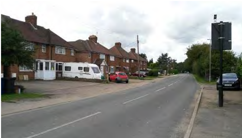
Figure 6.4 Residential properties along Denny End Road, particularly vulnerable to environmental effects of traffic coming in off the A10. Could be partly mitigated through high quality boundary treatment and street planting.
