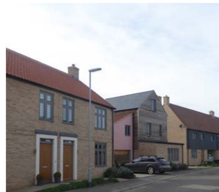
Fig. 68 - Artificial diversity, with mix of materials, colours and massing is in contrast with Fulbourn's simplicity
