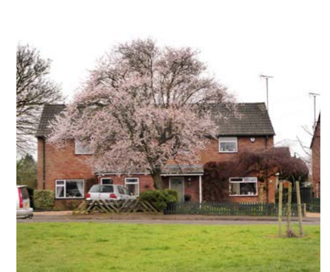
Fig. 38 - Strong front edge with walls and trees is typical of Fulbourn
