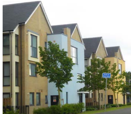
Fig. 64 - Taller frontages along a street are urban and out of place
