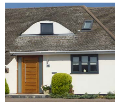
Fig. 36 - Upgraded doors and windows in contemporary style
