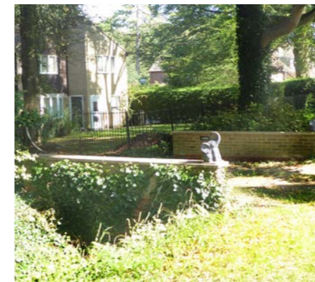
Fig. 21 - Drainage channels: a typical feature of this fen edge village (C)
