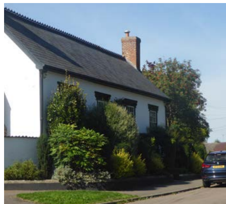
Fig. 52 - Planted street achieved without deep front gardens
