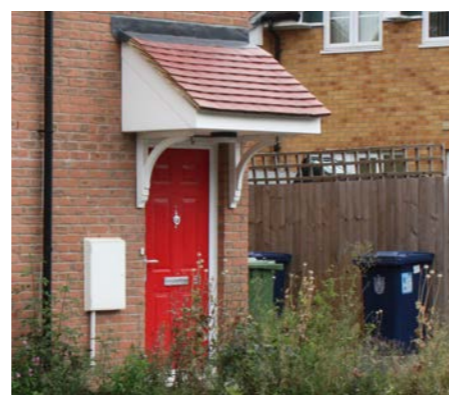
Fig. 73 - Prominent electric box and heavy porch details can spoil a facade
