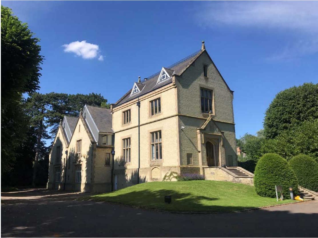
Figure 4: View of the Pump House facing north-east. A dense tree lined boundary surrounds the building.
