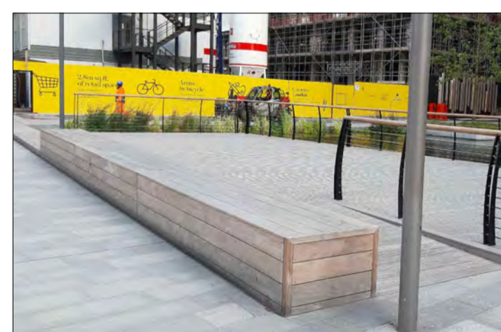
B2 Proposed Bench | Bespoke Bench | Fixing: As per manufacturer's specifications For details ref. to drawing TRF-CBA-1-GF-M2-L-8300
