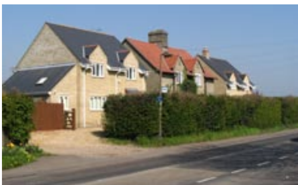
Nos. 9-11 Horningsea Road
