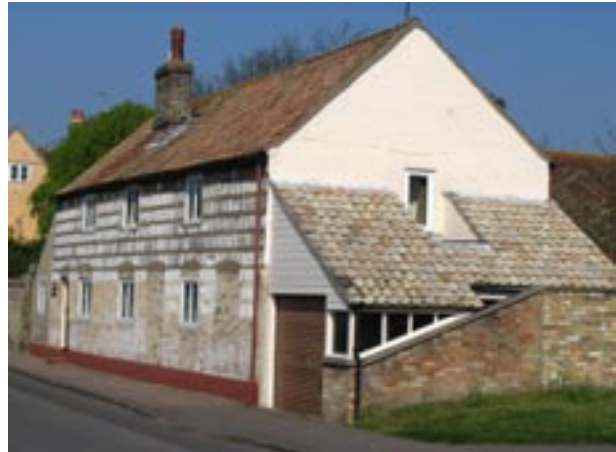
The Walled Cottage, No. 6 High Street
