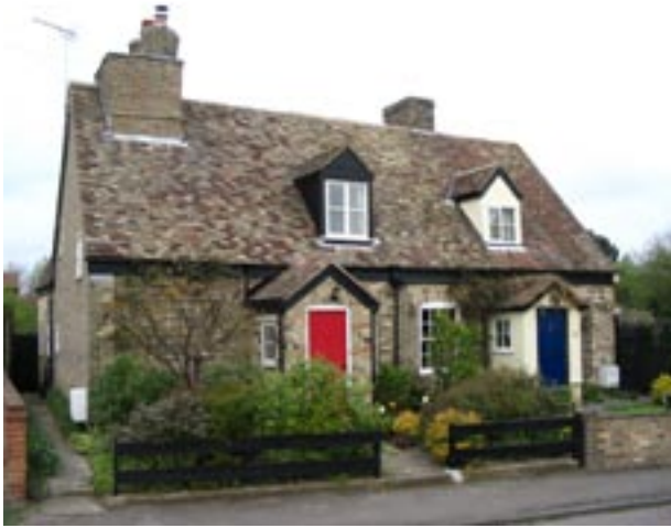
Nos. 1-3 High Ditch Road
