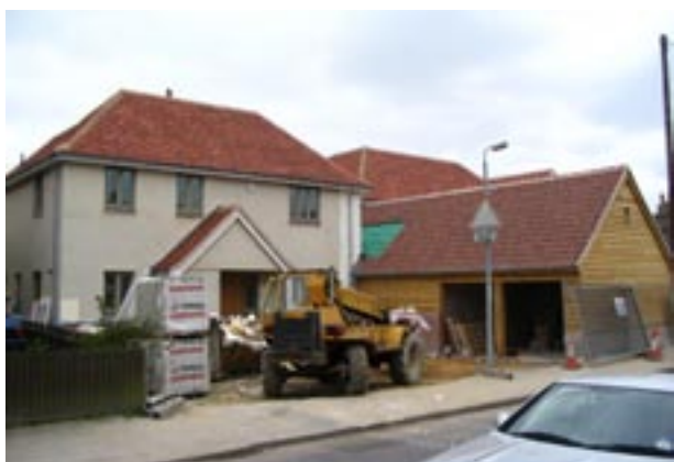
Nos. 8-10 High Ditch Road
