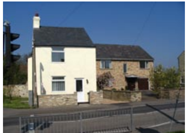
Nos. 1-3 Horningsea Road
