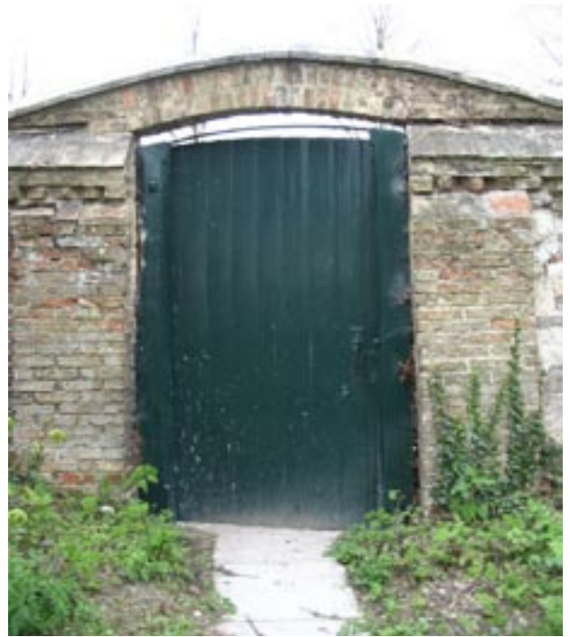
Gate in High Street wall to Ditton Hall
