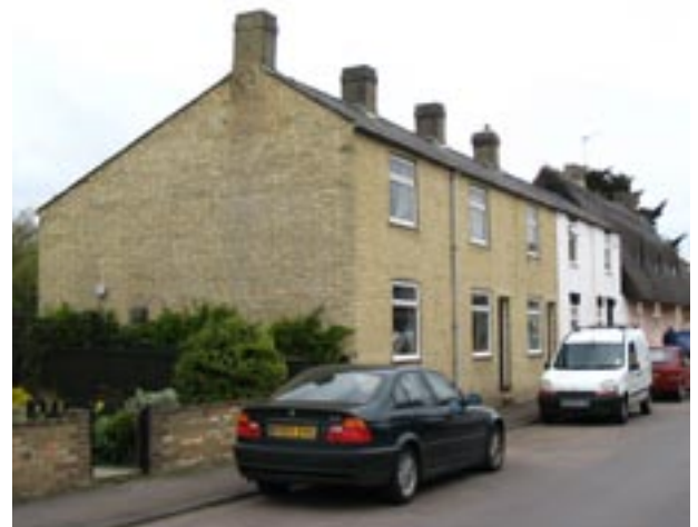
Nos. 5-13 High Ditch Road
