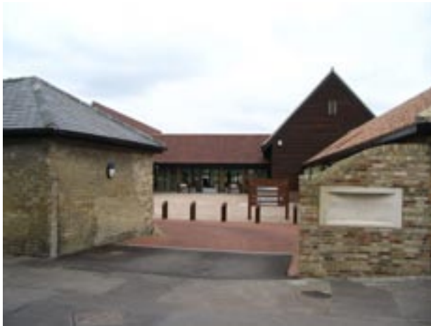
Francis Court, High Ditch Road
