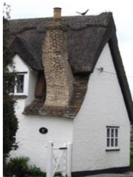
Chimney detail, No. 6 High Ditch Road
