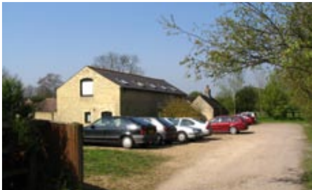
The Barn, Musgrave Farm
