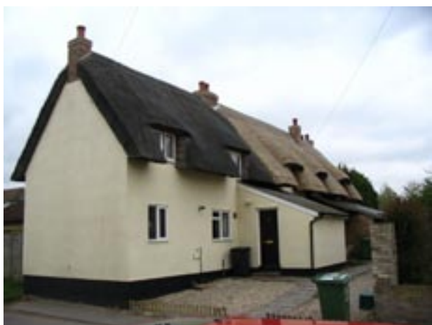
Nos. 14-16 High Ditch Road
