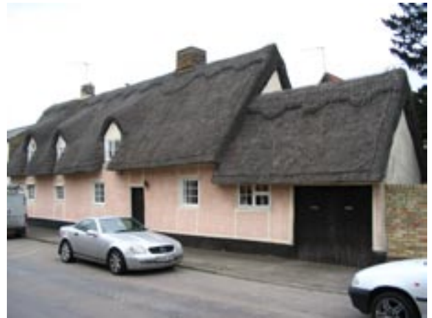
Nos. 15-17 High Ditch Road
