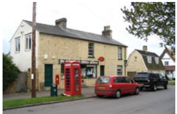
High Street Post Office with Listed telephone kiosk and No 17 beyond
