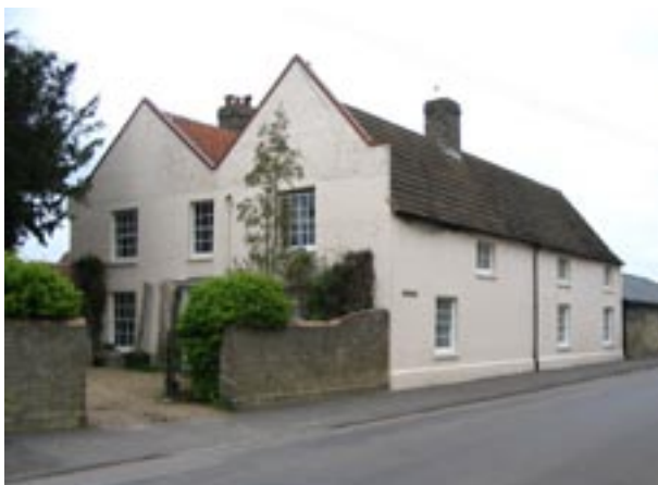
Mulberry House, No. 23 High Ditch Road
