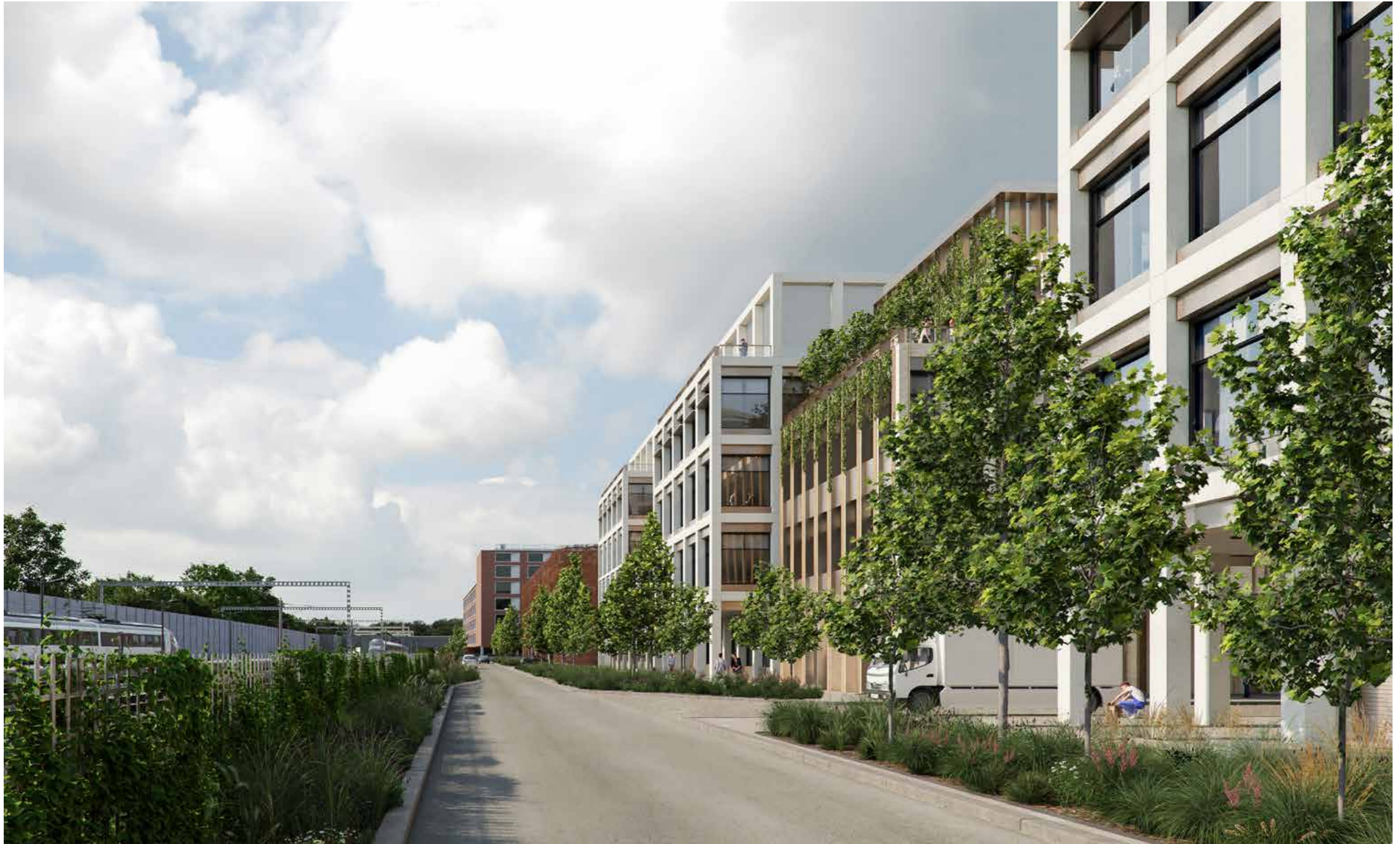
View looking south along Cowley Road along the eastern edge
