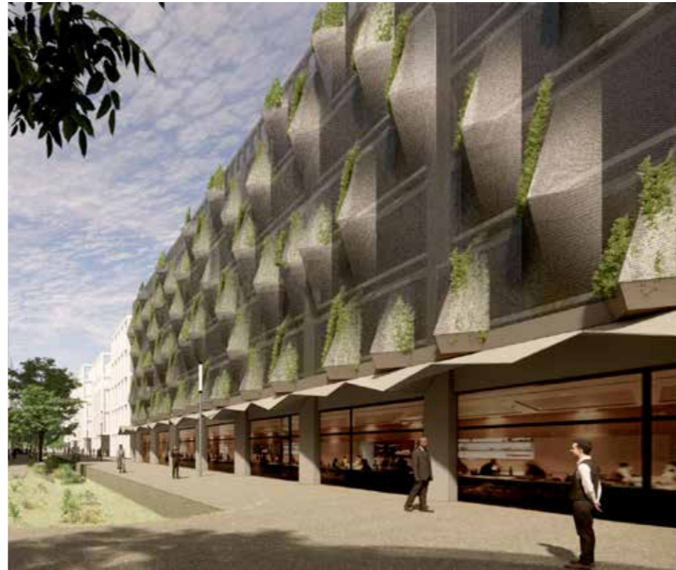
Mesh wrapped planters
