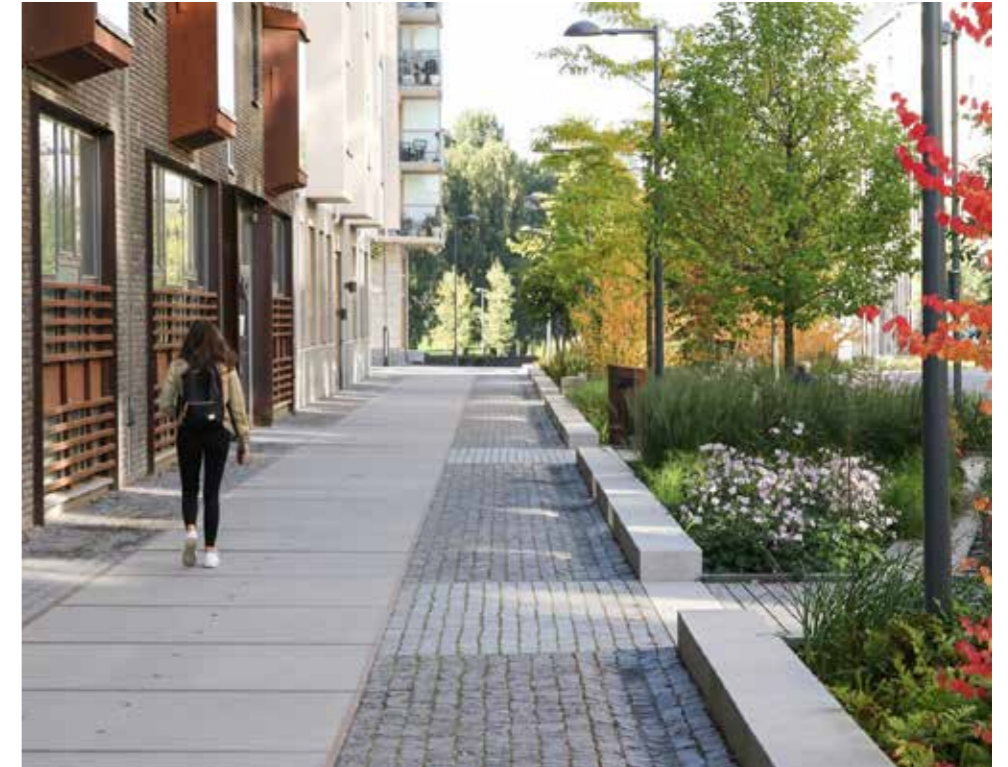
Chunky kerb with wide margin of granite setts
