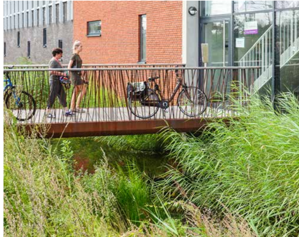
Narrow causeways to have visually permeable railing
