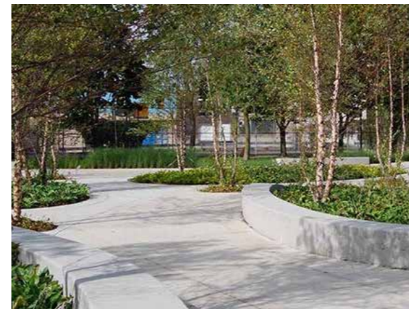
RAISED CONCRETE SEATING KERBS
