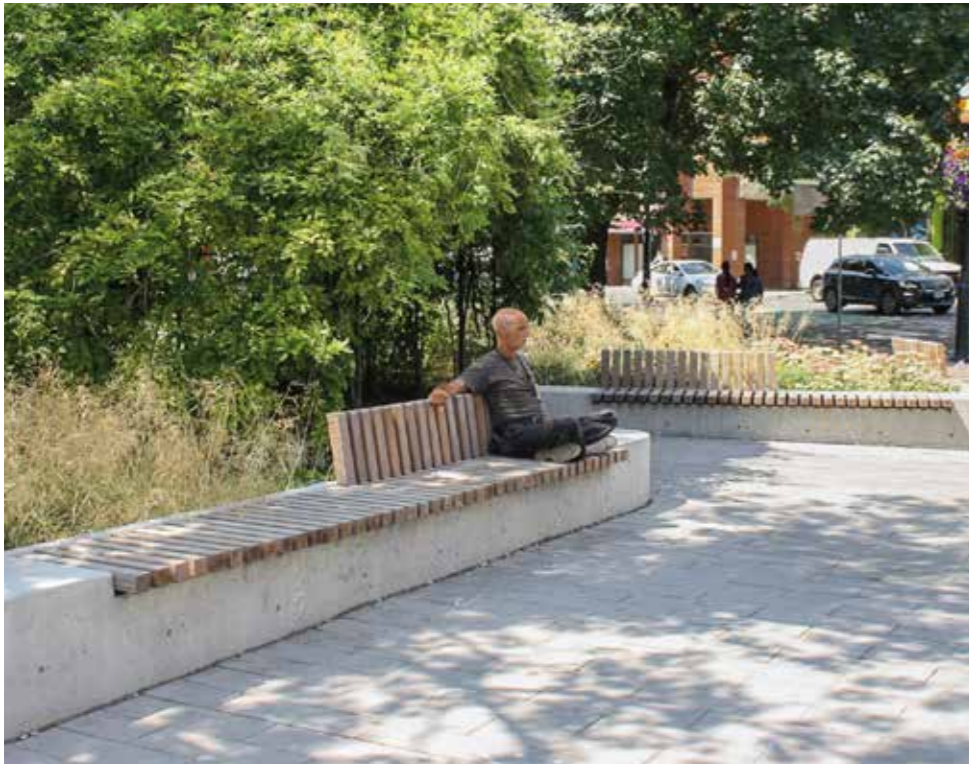
Hardwood timber slatted seating atop concrete base
