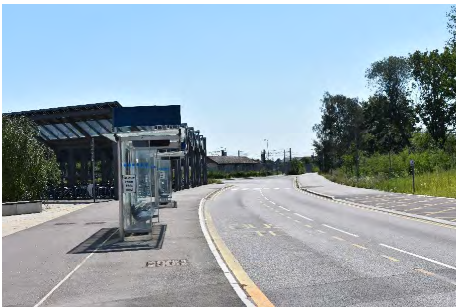
Figure 12.9: View South along the Cambridgeshire Guided Busway
