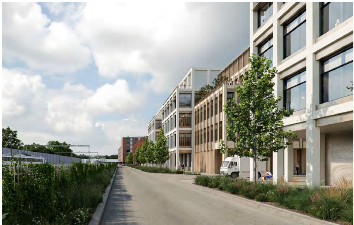
Figure 13.4: Architect CGI showing the material palette for the Proposed Development elevation fronting the rail tracks. These are mainly matte surfaces; some elements of the building are clad in metal and there are glazed areas.
