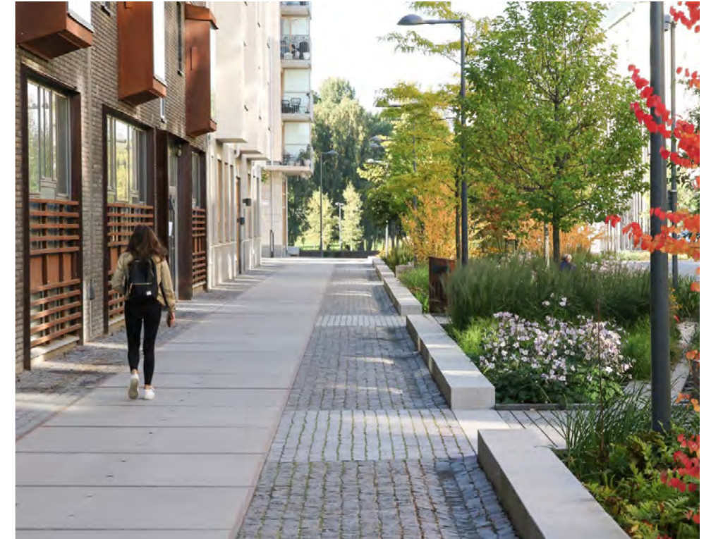
Chunky kerb with wide margin of granite setts
