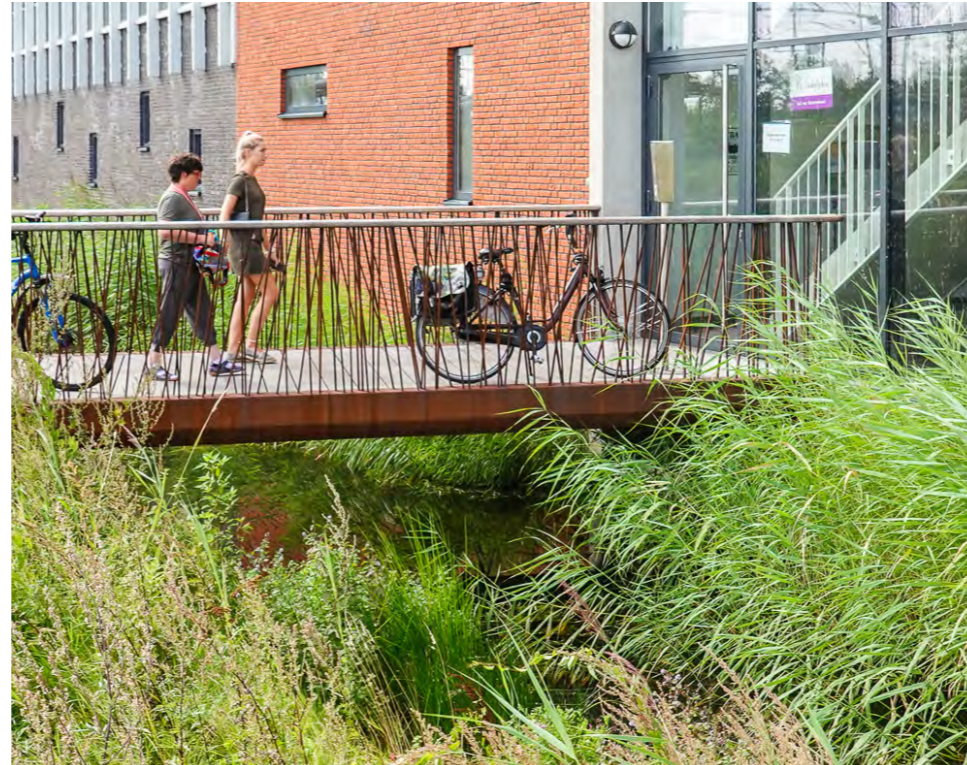
Narrow causeways to have visually permeable railing
