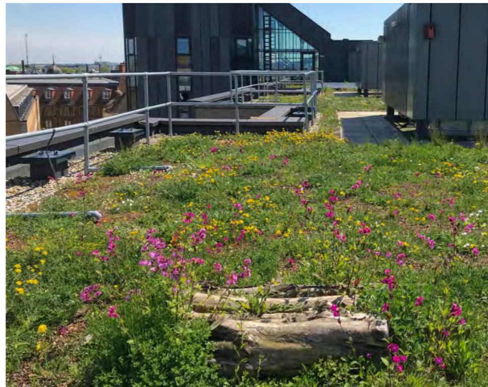
Deadwood piles and green roof seeding
