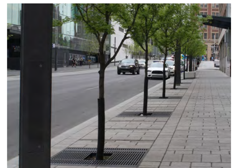
Trees in hard paving, to include underground root cells and underground guying
