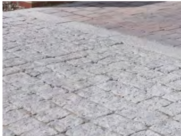
Granite setts, both flamed and tumbled
