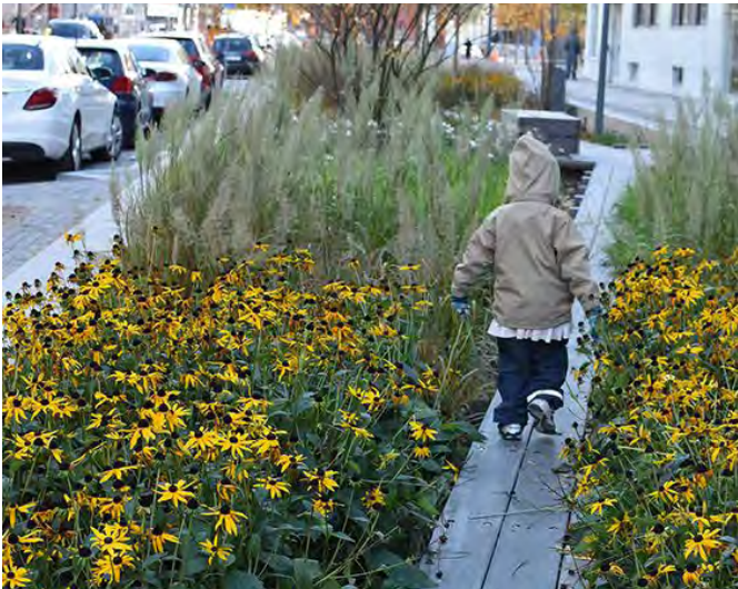
Fig.22 Timber planks crossing rain gardens
