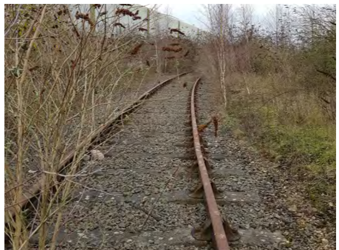
Fig.12 Site photo: Derelict railway infrastructure
