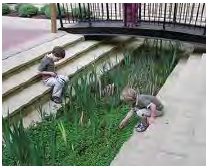
Fig.20 Linear SUDs feature with steps for up-close encounters
