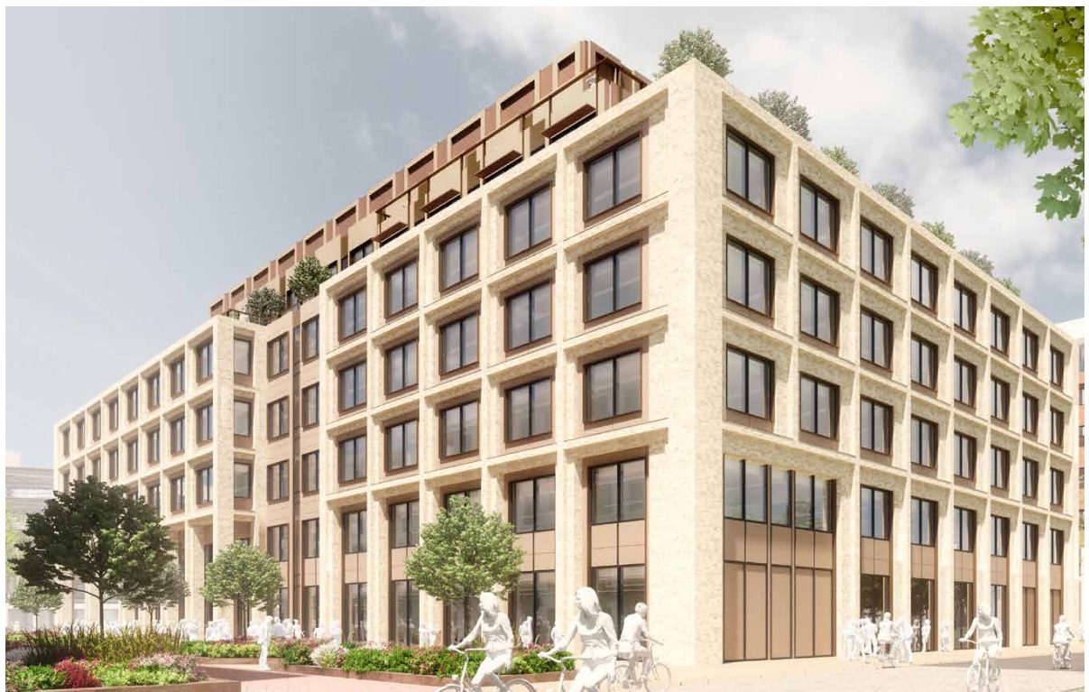
Figure 14 Illustrative view of S4 Milton Walk and Chesterton Way corner
