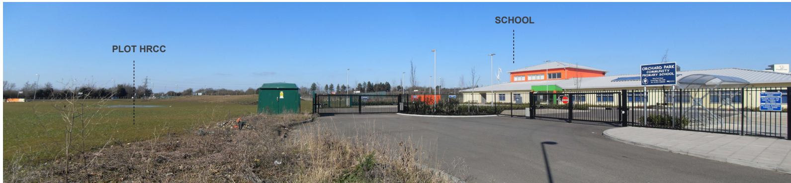
FIG 10 - PANORAMIC VIEW LAND PARCEL Q/HRCC LOOKING NORTH WEST TO SCHOOL
