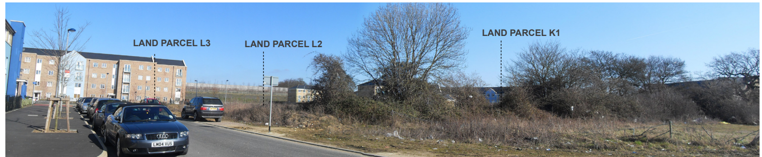
FIG 12 - PANORAMIC VIEW LAND PARCEL K1 LOOKING NORTH
