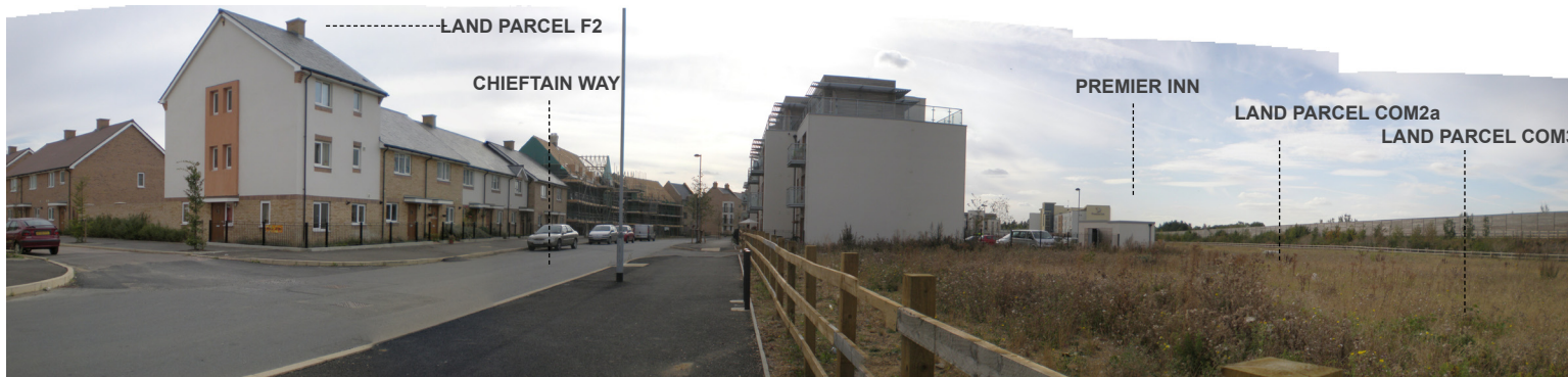
FIG 4 - PANORAMIC VIEW LAND PARCEL COM2b LOOKING WEST
