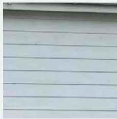
Weatherboarding timber painted white
