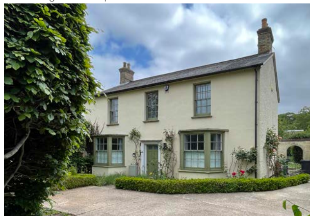
Figure 78: Creamy render facade with recessed porch in olive green. Sash and bay windows with olive green painted frames.
