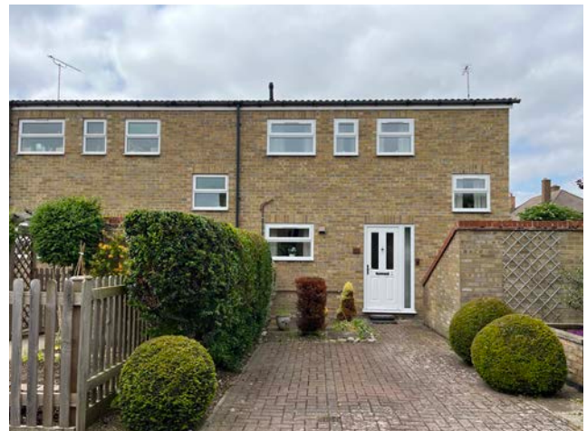
Figure 65: 2 storey semi-detached houses with buff brick
