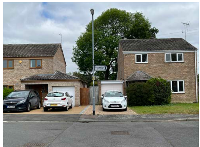
Figure 54: Detached houses with buff brick. The one to the left presents a side and front extension
