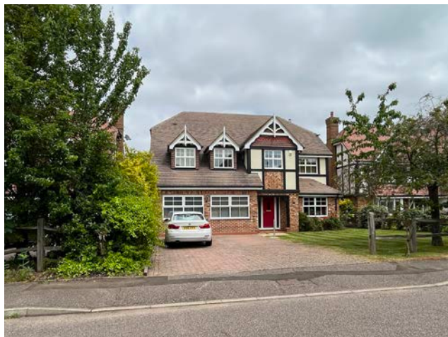
Figure 58: Large size detached house in red brick and render with decorative timber elements and dormer
