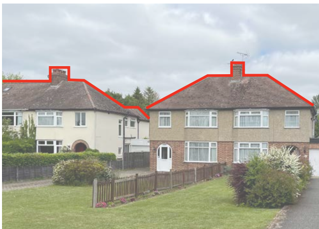
Figure 68: Example of hipped roofs along London Road
