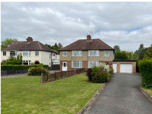
Figure 57: Well set back semi-detached housings, 2 storeys with hipped roofs
