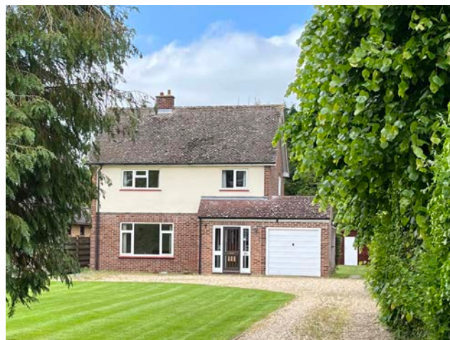
Figure 48: Detached house with pitched roof
