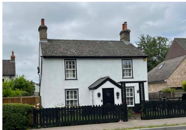
Figure 77: White render and black sash window frames. Protruding enclosed porch.
