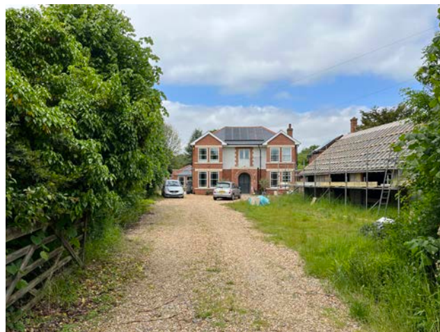
Figure 46: Well set back house with high hedgerow to the left
