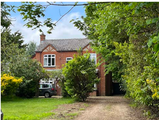
Figure 45: Well set back detached house with high hedgerow to the right and a landscaped front garden
