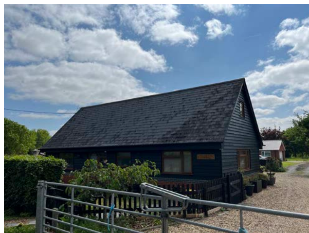
Figure 17: Parkfield converted commercial building
