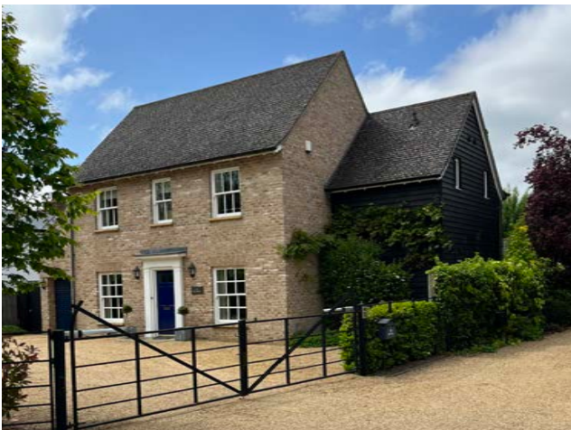
Figure 38: Detached house in buff Cambridge brick with side extension in timber
