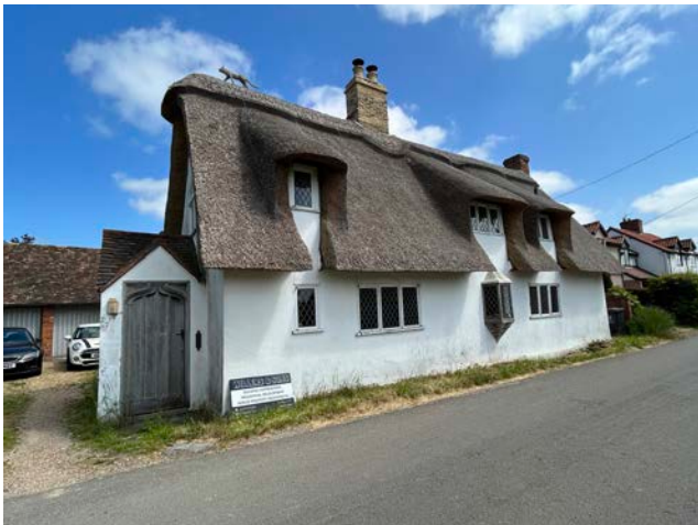
Figure 13: Hope Cottage, 2 storeys with thatched roof
