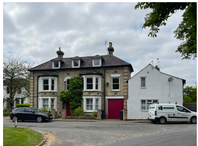
Figure 24: Melbourn House, 40 Royston road. 3 storeys house with dormer windows; Cambridge brick with some ornate brickwork from 1870s and bay windows
