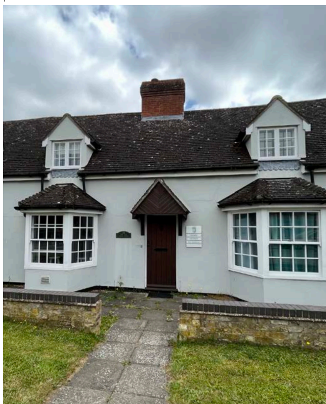
Figure 74: Porch, sash, bay windows and dormers
