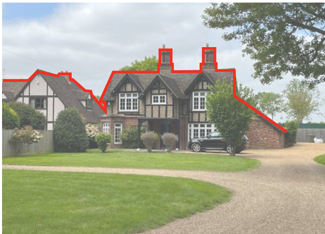
Figure 67: Example of varied pitched roofs on the High Street
