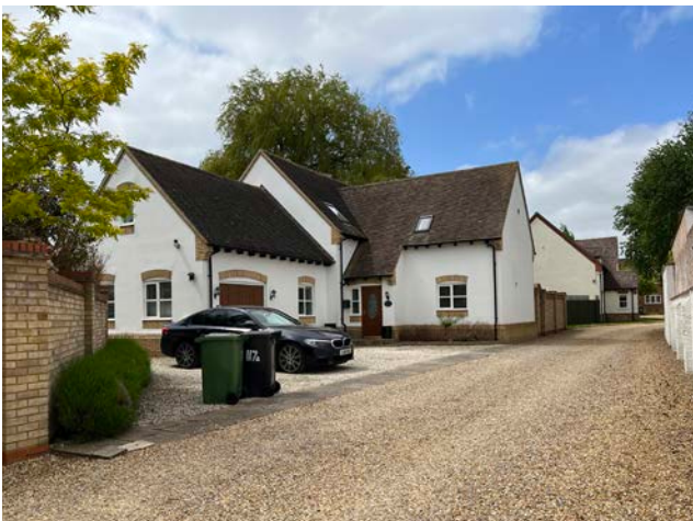
Figure 39: Detached house with varied roofline in white render and decorative elements with buff brick
