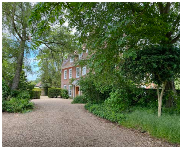
Figure 03: Harston House and Part of Garden Wall, Grade II* listed building.
