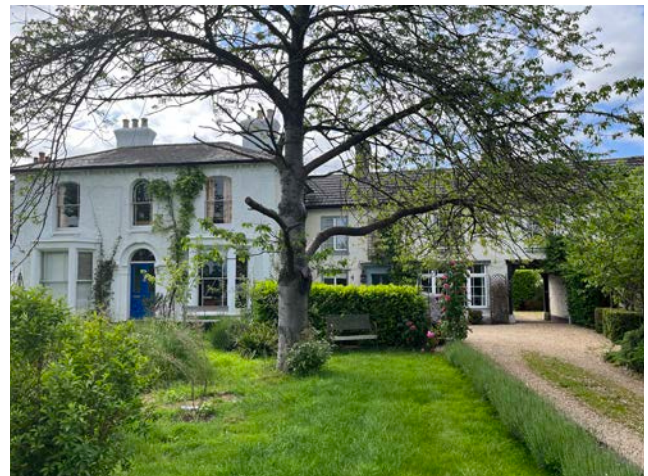
Figure 23: Semi-detached 2 storey buildings with deep front gardens
