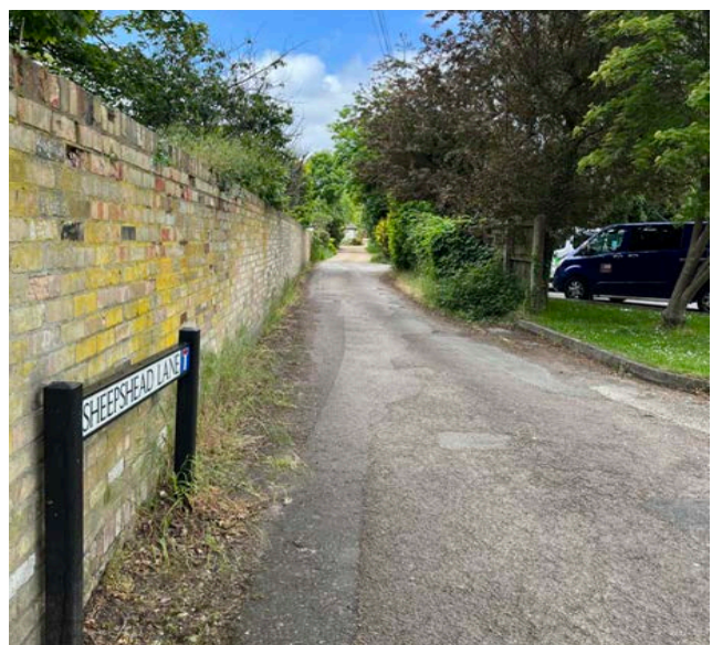
Figure 85: Narrow lane in tarmac
