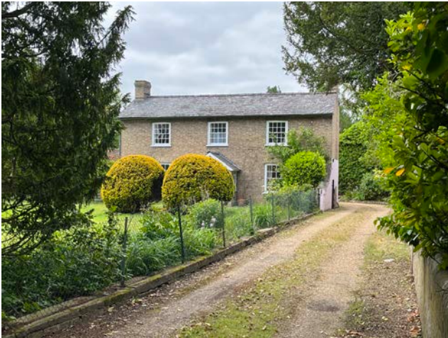
Figure 37: Detached building with buff brick and manicured front garden
