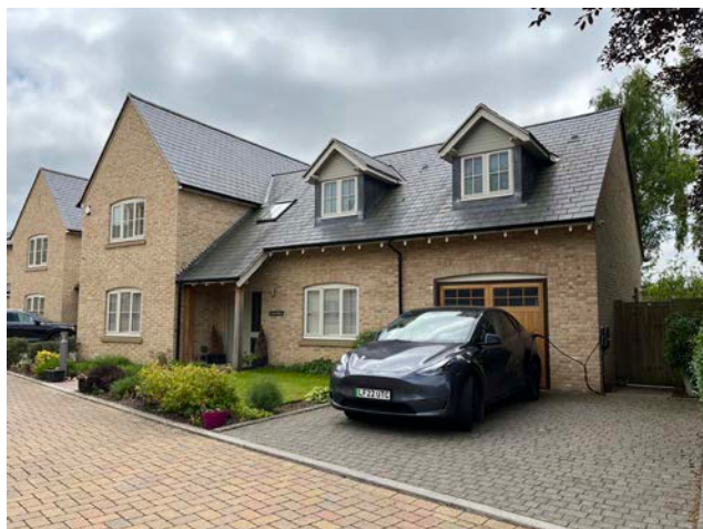
Figure 60: The Pastures. New development using traditional materials
