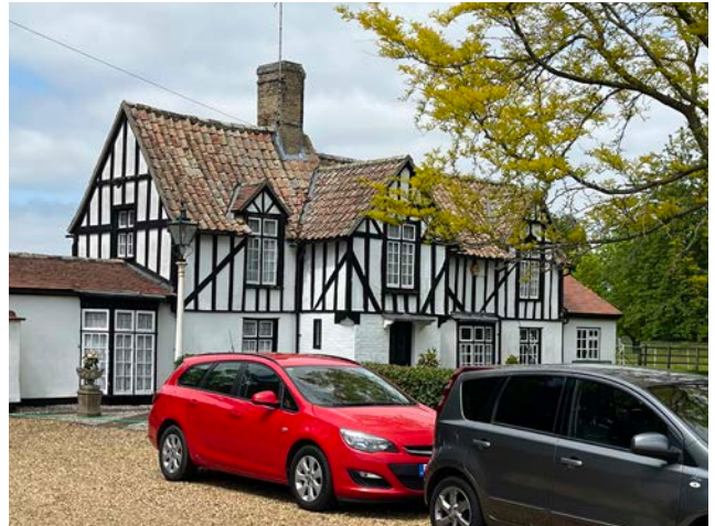
Figure 28: White rendered building with timber structure and pitched roof
