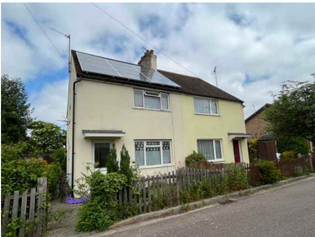
Figure 62: 2 storey semi-detached houses with narrow front garden
