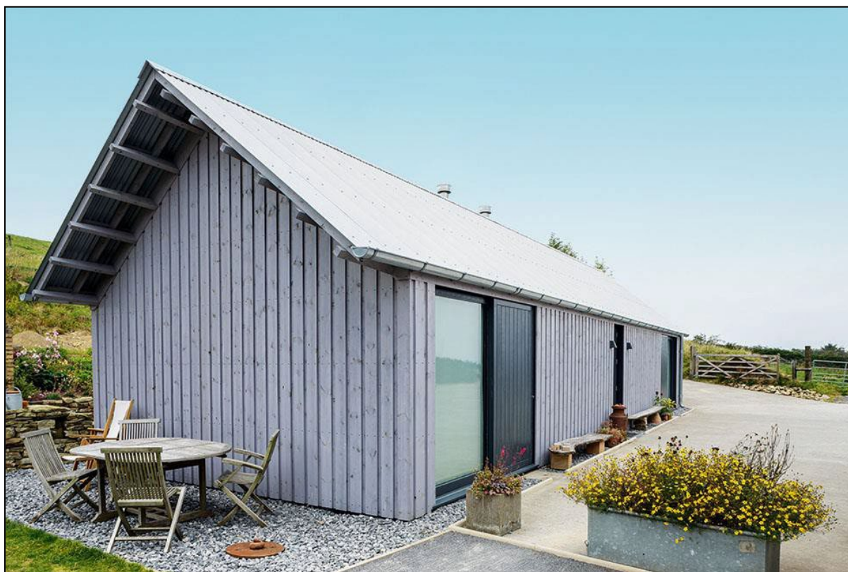
An example of a small single storey, affordable and secure barn style building 78
